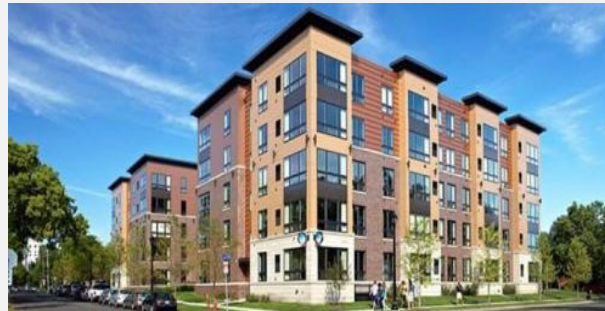
412 Lofts – University of Minnesota, Minneapolis, MN
