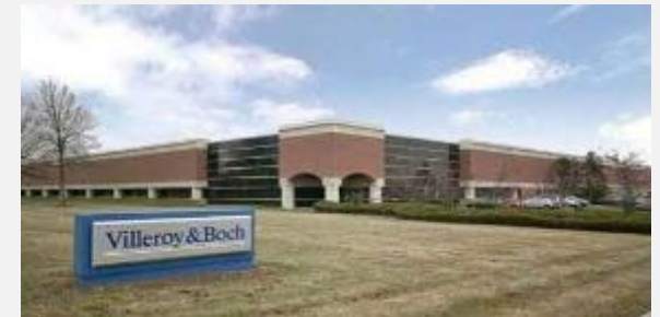
3 South Middlesex Avenue, Monroe, NJ
