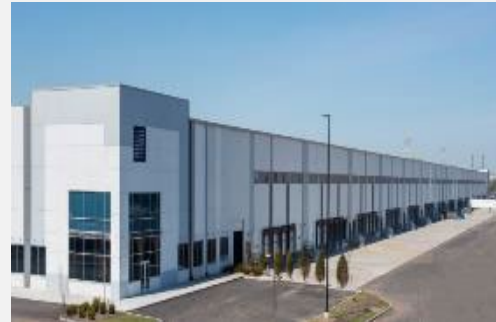
586 Gulf Avenue, Staten Island, NY
